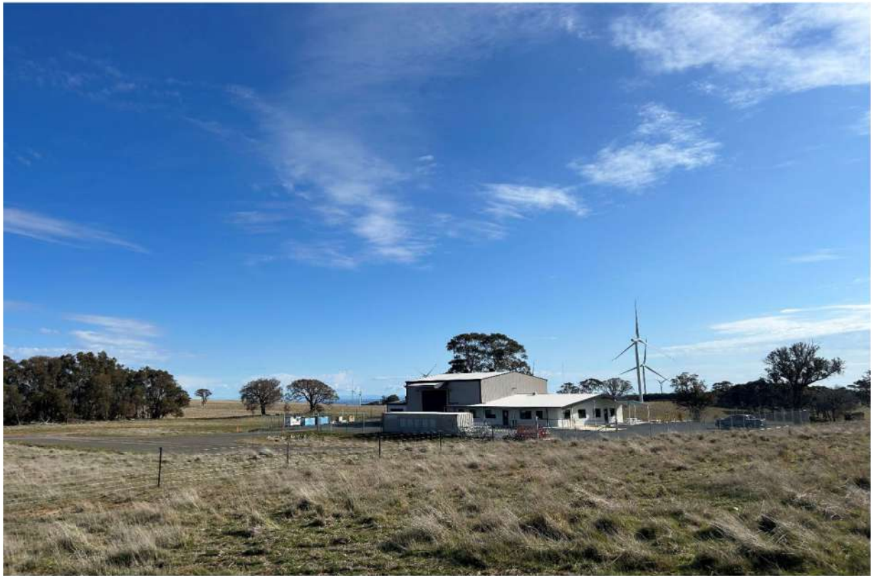
Plate 7 – O&M building from entry road
