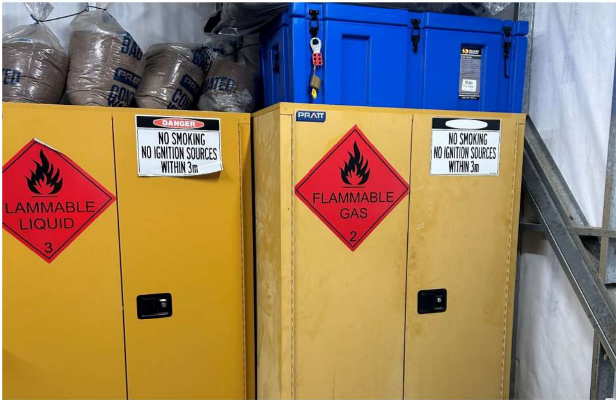
Plate 3 – Flammable liquid storage within storage shed
