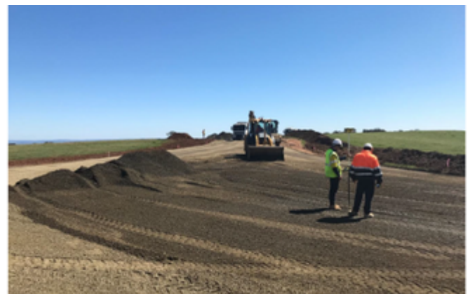
Gravelling the Intersection
