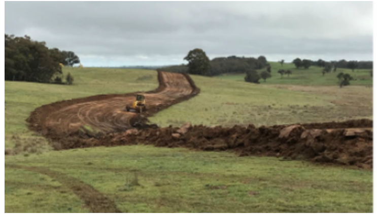
Stripping soil for access tracks
