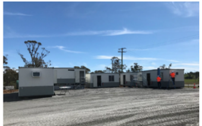
Buildings installed in the compound
