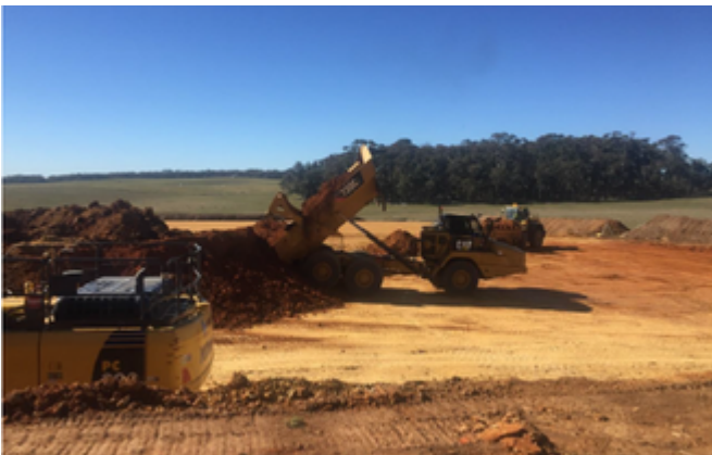
Earthworks for temporary work compound
